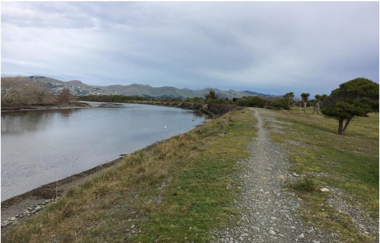
Figure A4 – 11 July 2017 existing stopbanks on true right bank of estuary approximately point 9840 on C229 looking south. Proposed works including topsoiling and landscaping to raise the height of the stopbank by 0.06-0.54m.
