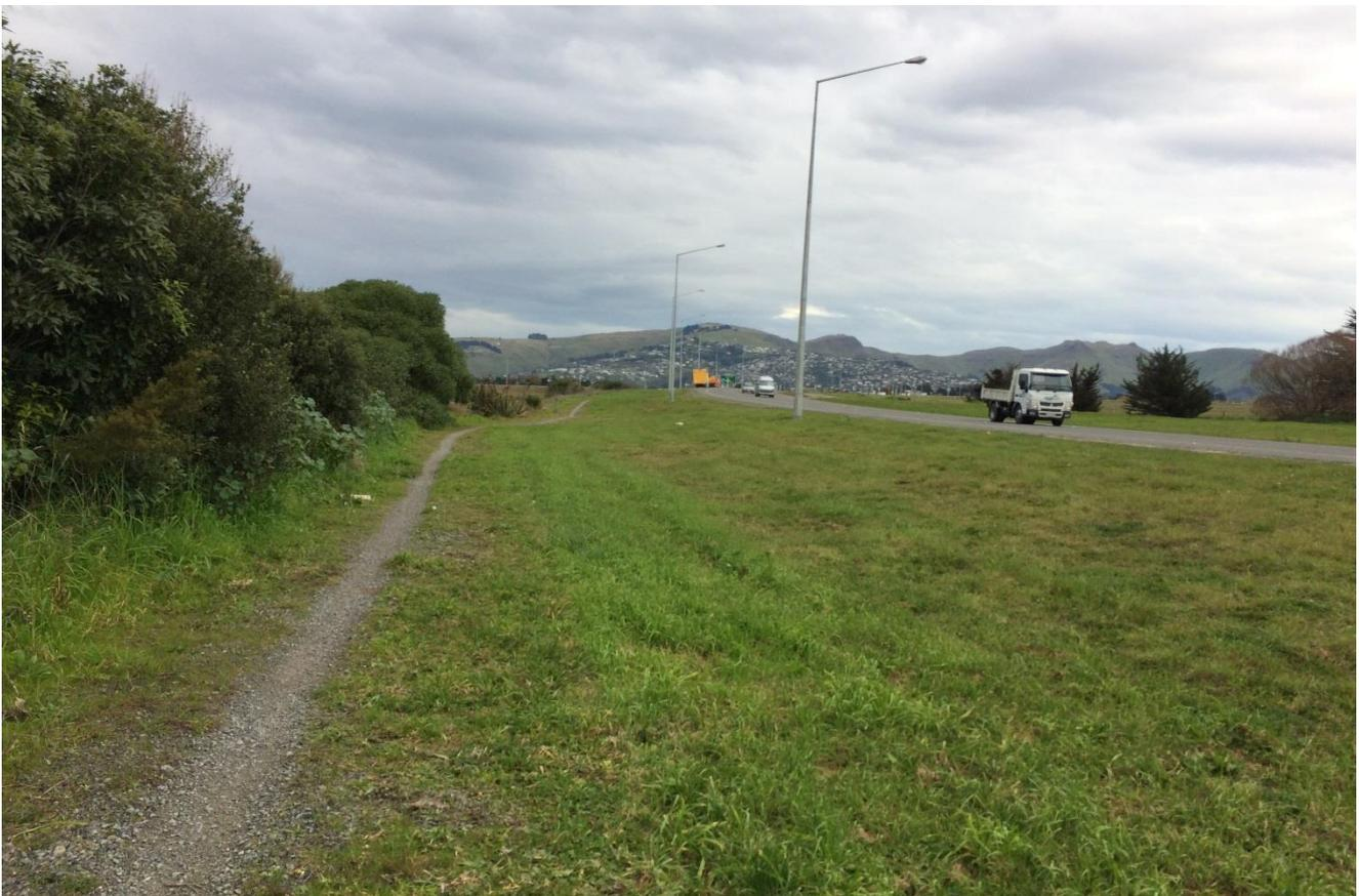
Figure A22 13 June 2017 Location of proposed temporary stopbank on east side of Bexley Road looking south. Bexley Road on right. Stopbank to be built over the existing gravel path increasing the height between 0.0 and 0.37m.
