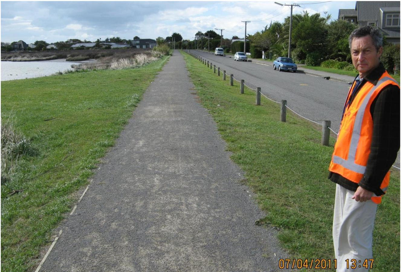
Figure A9 – 7 April 2011 – Kibblewhite Street looking north from approximately point 10420 on Plan C131 showing height of stopbanks post-earthquakes but before emergency works
