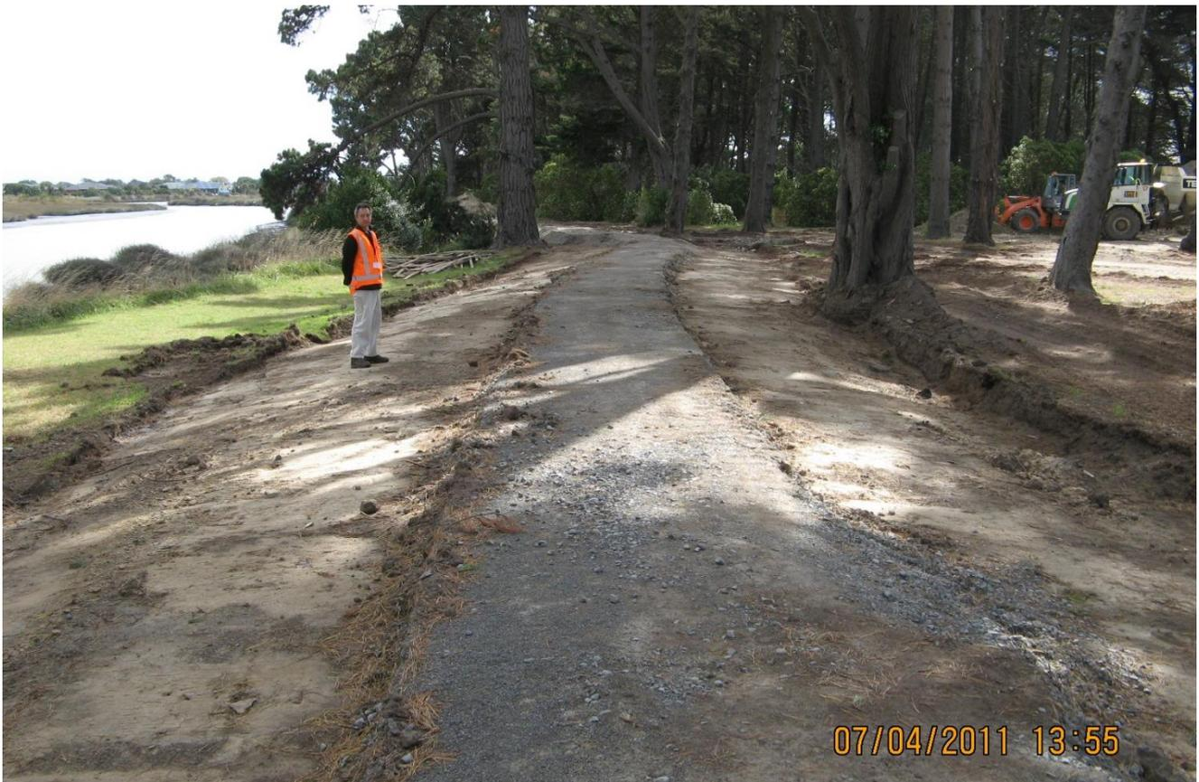
Figure A3 April 2011 – Blighs Garden preparation for installation of stopbank (approx. between points 9760 and 9980 on Plan C129) showing level of pathway post-earthquakes but pre-emergency works.
