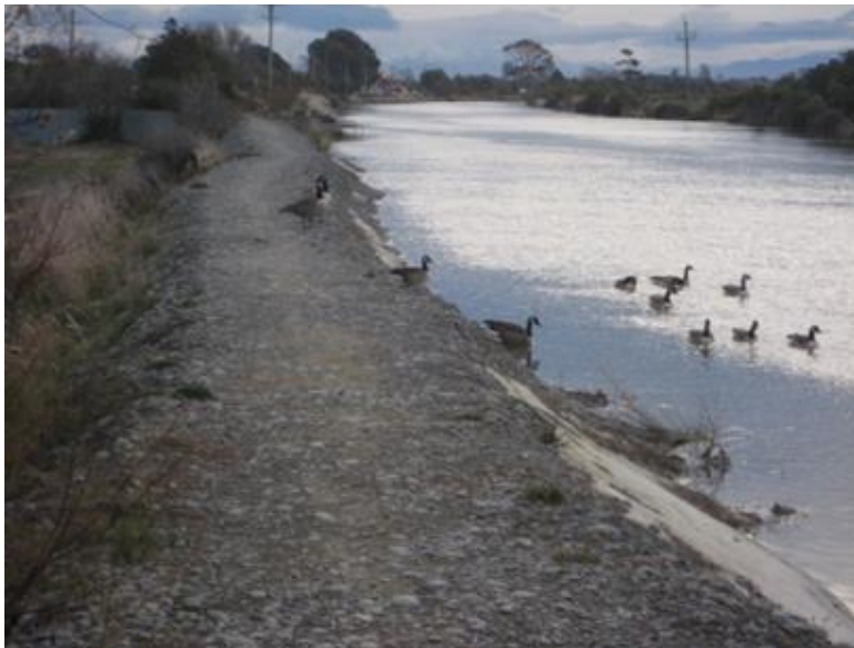
Figure 3-23 Section 17 Right Bank – Typical gravel fill Stopbank
