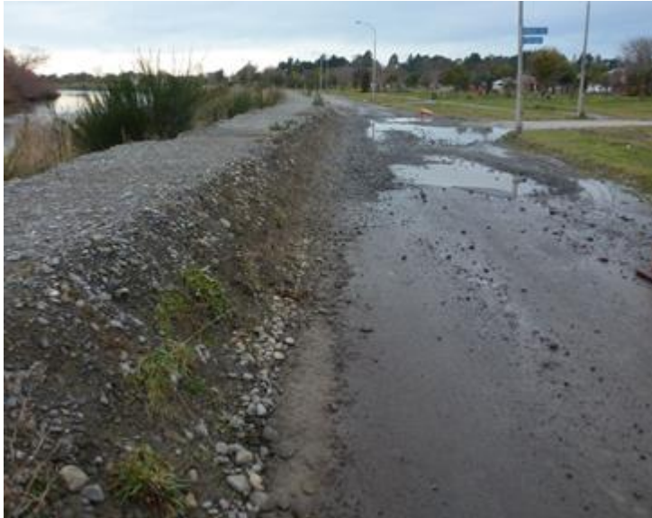
Figure 3-6 Photograph of Typical Levee Section 15
