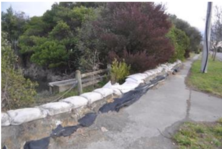
Figure 3-24 Section 6 – Left Bank – Example of Sandbags
